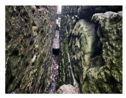
High external ground level between right hand gable and boundary wall
