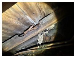
Decay to rafter and adjacent sarking to apex void
