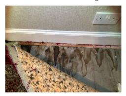
Staining and high moisture readings to floorboards adjacent to right hand wall to ground floor room right
