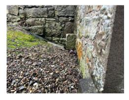
High external ground level to rear elevation
