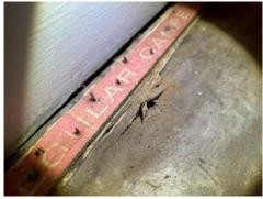
Decay to floorboards to rear of ground floor room right
